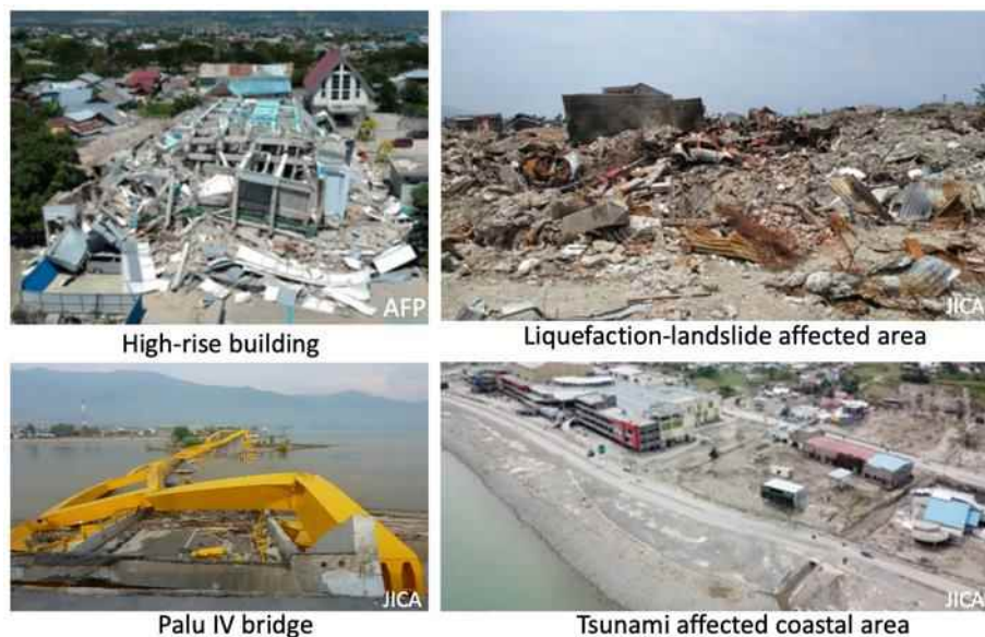
Fig. 6.1 Damaged buildings and facilities
