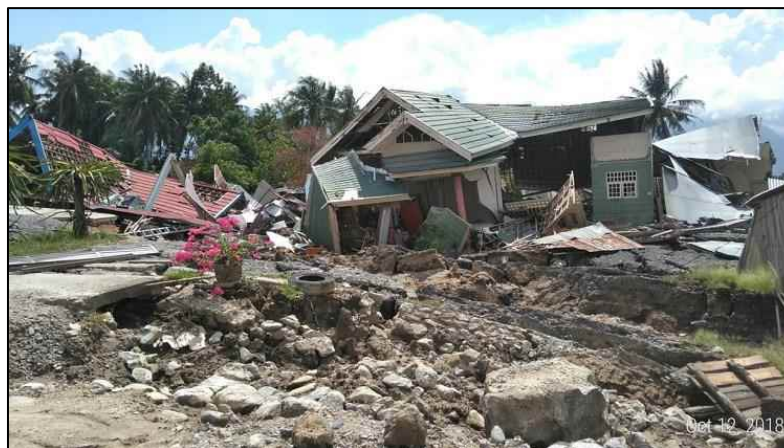
Figure 7.9 Collapsed House in Balaroa
