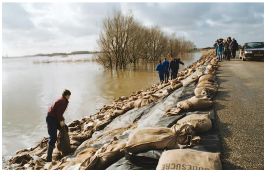
Figure 10.4 Emergency repair during high water at Ochten, The Netherlands in 1995
