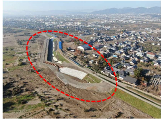
Fig.4.4 Emergency restoration work at Chikuma River (Double-wall pile sheeting coffer dam)
