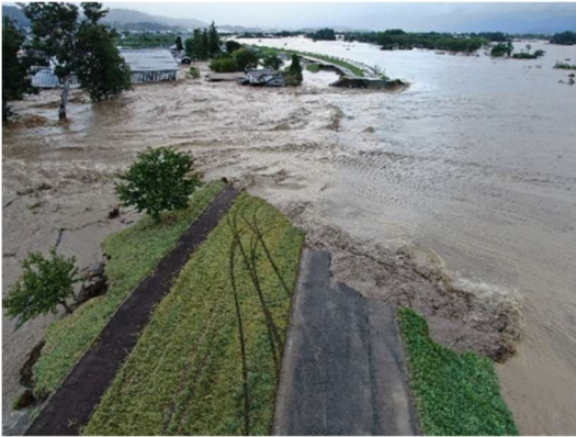
Fig.4.3 Levee Breach at Chikuma River
