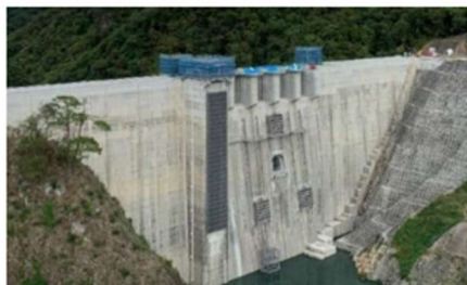
Yamba Dam before & after water storage
