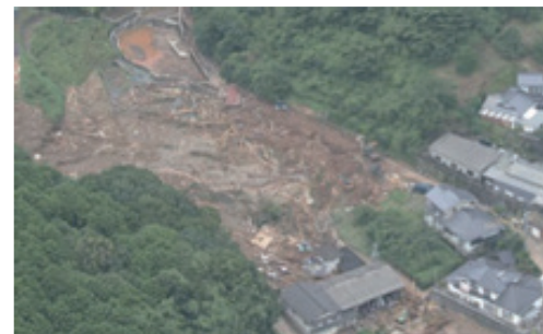
Damage due to debris flow (Tsunagi-cho Fukuhama, Ashikita-gun, Kumamoto)
