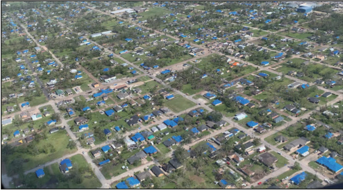
Figure 6. An aerial photo shows some of the more than 8,000 blue roofs that were installed after Hurricane Laura that survived Hurricane Delta just a few weeks later – approximately 87% of all USACE-installed roofs survived the second storm.
