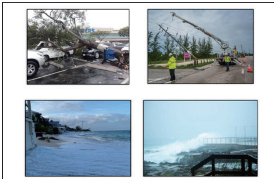
Figure 6. Showing the damages of Tropical Storm Eta in the Cayman Islands, November 2020. Source: CCRIF SPC Event Briefing for Tropical Cyclone Eta, November 18, 2020.
