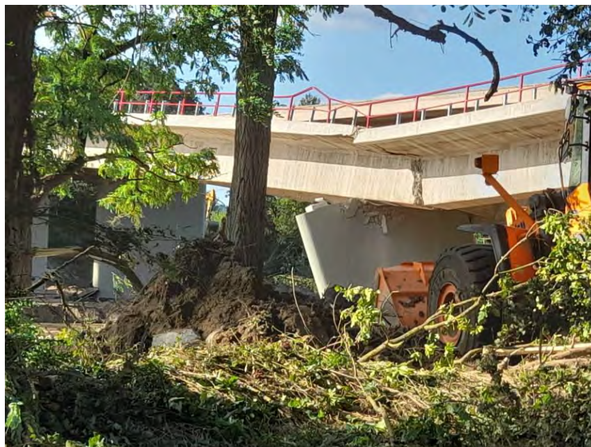
Figure 10: Destroyed bridge in Sinzig (Photo Peter. Ruland)
