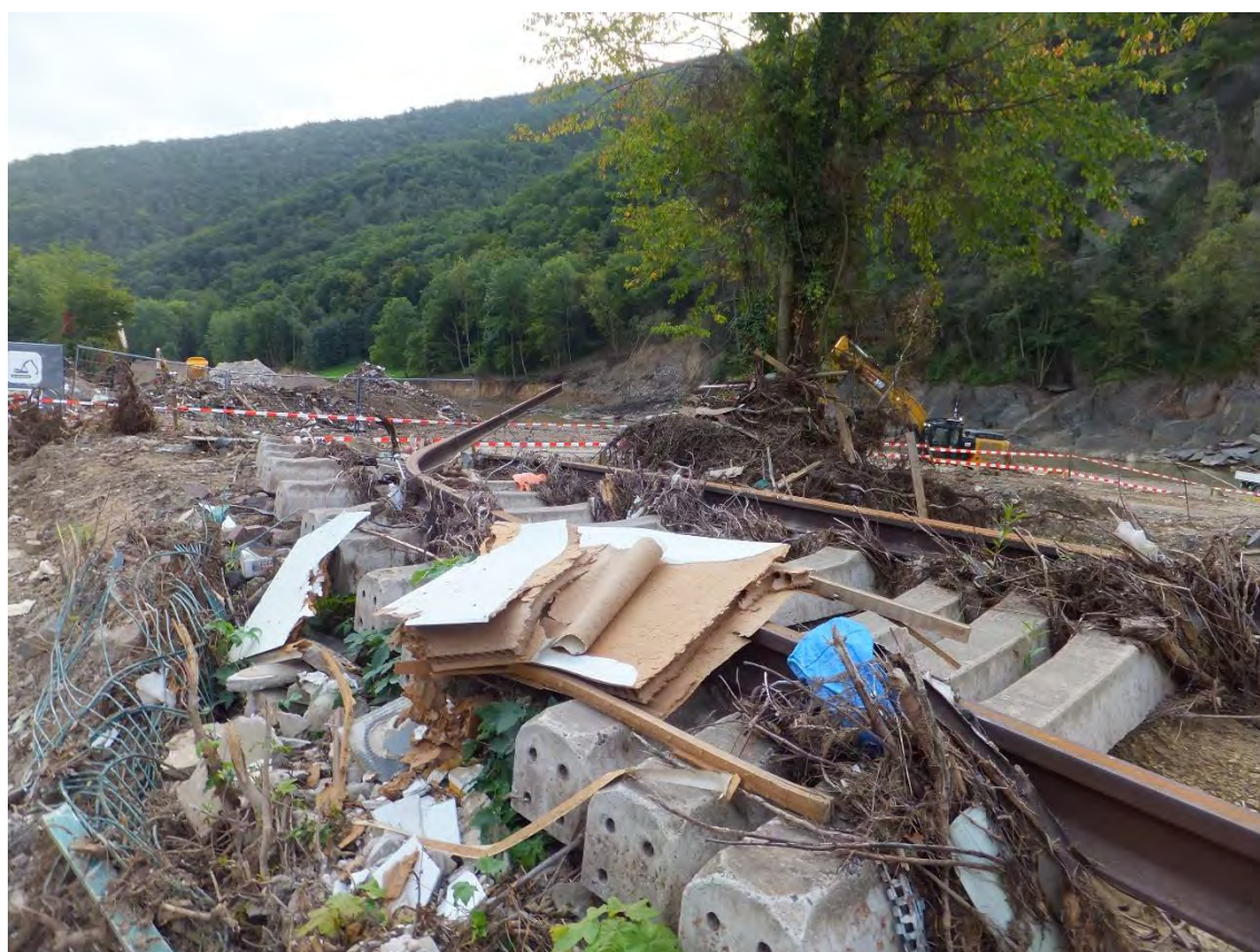
Picture 1.1 Damage to railway along Ahr River by Heavy Rain Disaster in Germany in July, 2021
