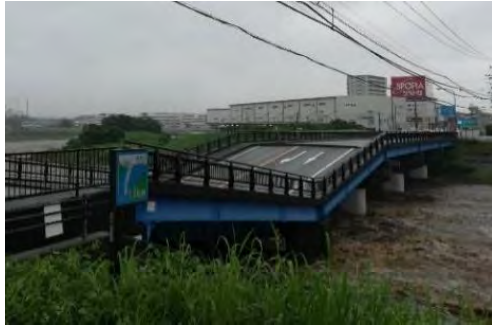
Overflow and Inflow (Rokkakugawa River)
