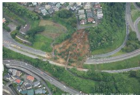
Slope collapse at Zushi Interchange (Zushi City, Kanagawa Pref.)
