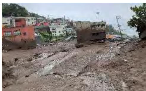
Damage caused by Mudslides (Atami City, Shizuoka Pref.)
