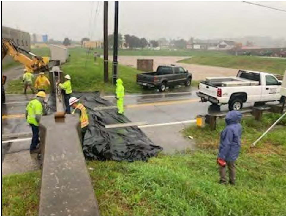
Figure 7. USACE Baltimore District team members and contractors install road closures Sept 1, 2021, in York, Pennsylvania, ahead of Ida's arrival. (U.S. Army photo)
