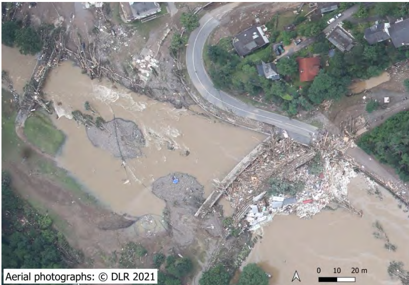
Figure 8: Accumulation of debris at a bridge near Altenahr (DLR 2021)
