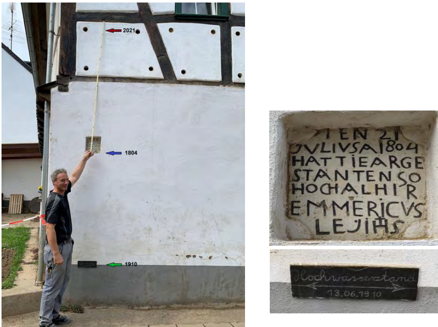
Figure 7: Water marks in Walporzheim: The 1910 mark is about 50 cm above the ground level; the 1804 mark is 1.7 m higher and the 2021 mark 3.5 m higher than the flood level in 1910. The 1804 flood is remembered by an inscription “Ten 21 Julius a(nno) 1804 hat tie ar gestanten so hoch alhir Emmericus Lejihs” - “(On) the 21 July 1804 has the Ahr stood so high here. Emmericus Lejihs (owner)”. 1910 is remembered by “Hochwasserstand (flood level) 13.06.1910” (Photo A. Fekete)
